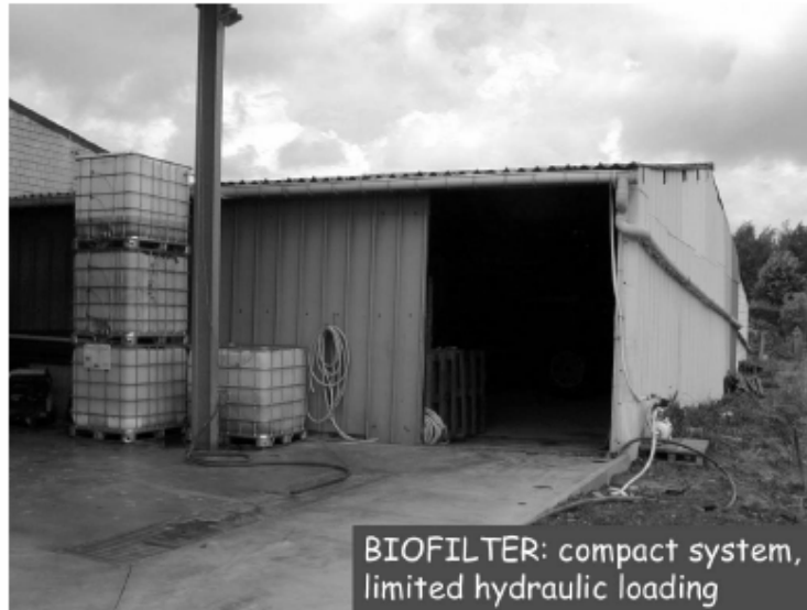
Fig. 22. Modified biobed-filter with stacked serial filter units (Jaeken & Debaer, 2005)
